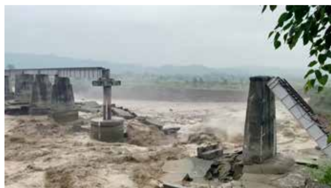
A general view of a bridge that collapsed following heavy rains in Kangra, Himachal Pradesh, India
